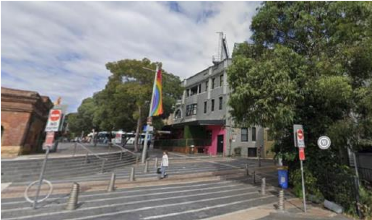
Figure 12: Rear of sign structure as viewed from Bourke Street (Google Streetview)
